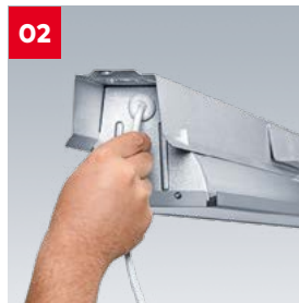
02 Bring the cable through the cable entries on the side or top of the housing
